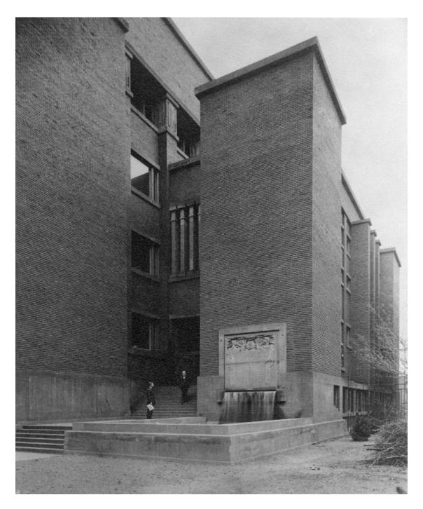
Since the building was surrounded by coal-burning trains and smoke-belching factory chimneys, a major objective was to not only control temperature within the building but provide clean air. So, air from the outside was pumped into the towers where it went through a cold water spray and filter, then heated to the desired temperature before being discharged into the interior.
